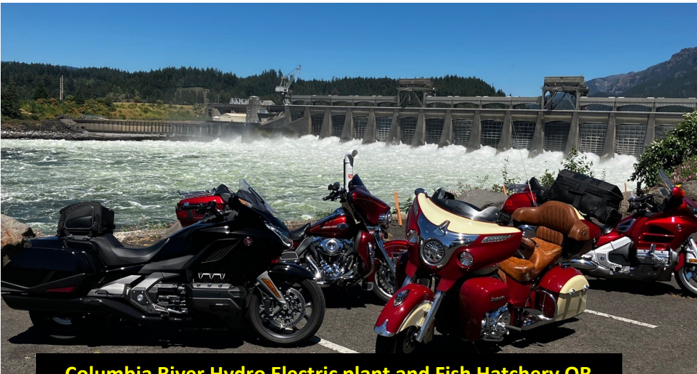
Columbia River Hydro Electric plant and Fish Hatchery OR
